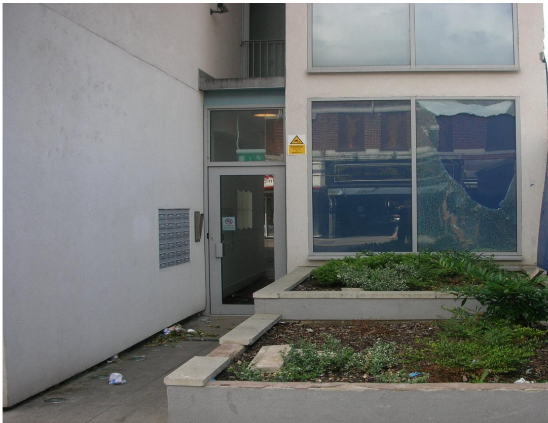
Poor design and location of main communal entrance, lacking natural surveillance and supervision.
