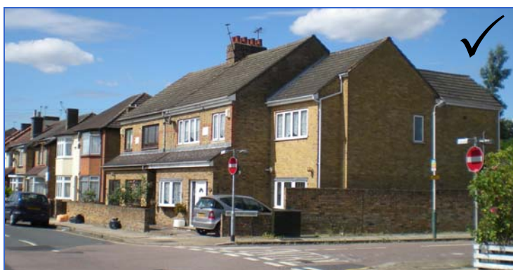
Figure 12 Combined side and rear extension to corner property
