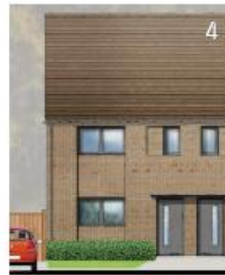
4 Removing overhanging eaves and fascias and replacing with clipped verges and rise and fall gutter brackets; rainwater goods in grey
