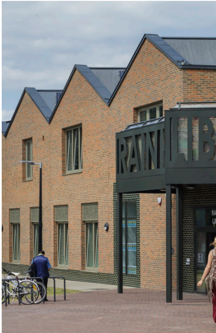
Rainham Library, Maccreanor Lavington Architects © Tim Crocker
