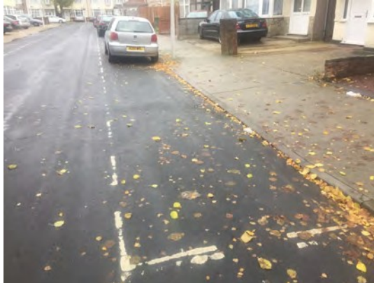
Many marked out Residents Permit Holder spaces cannot be parked on as the block private driveways (Zones 1,2,4, 5 and 6)
