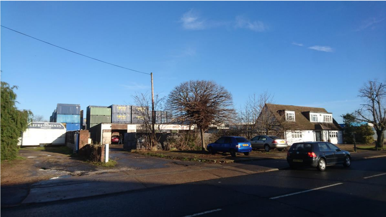
View towards Site from Crow Lane
