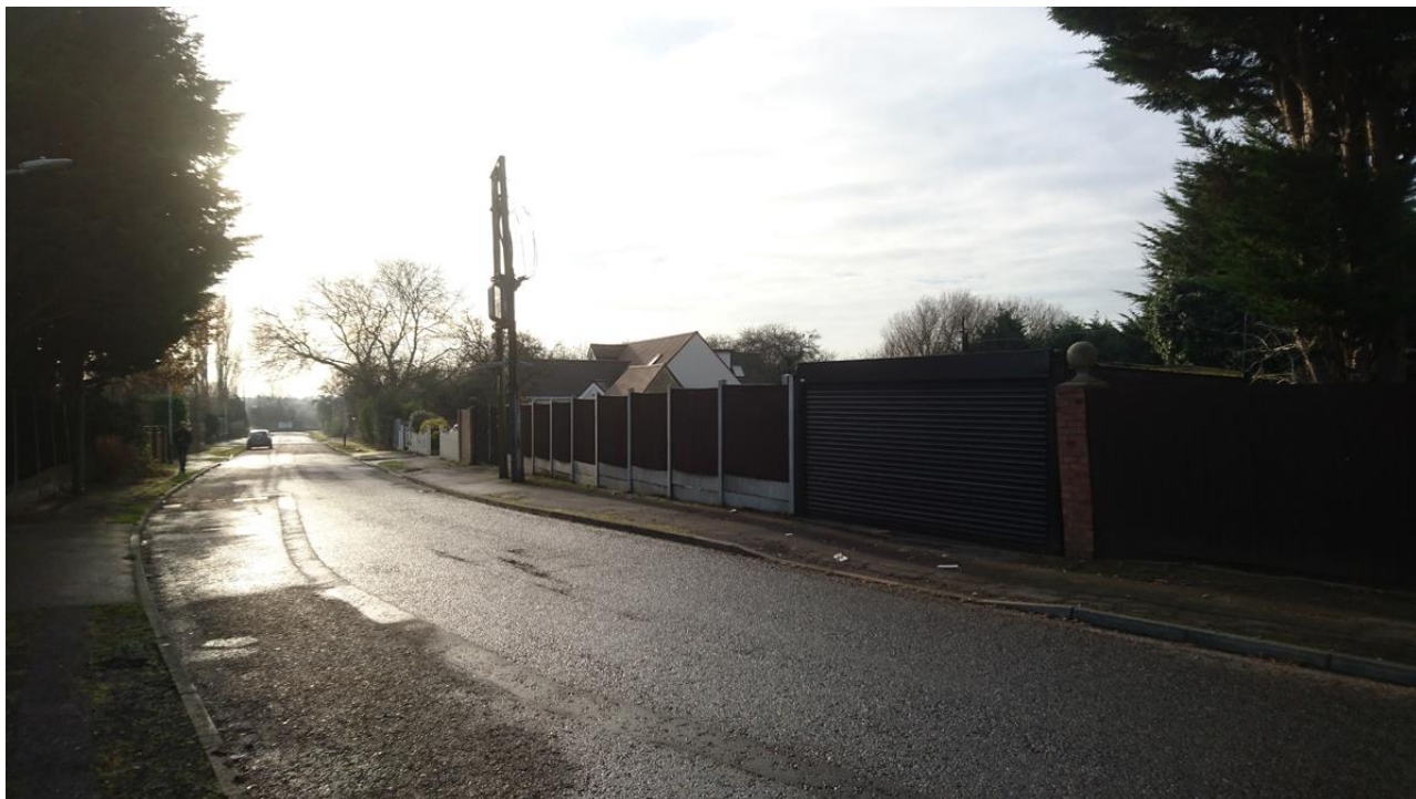
View of Site's eastern Boundary from Risebridge Chase
