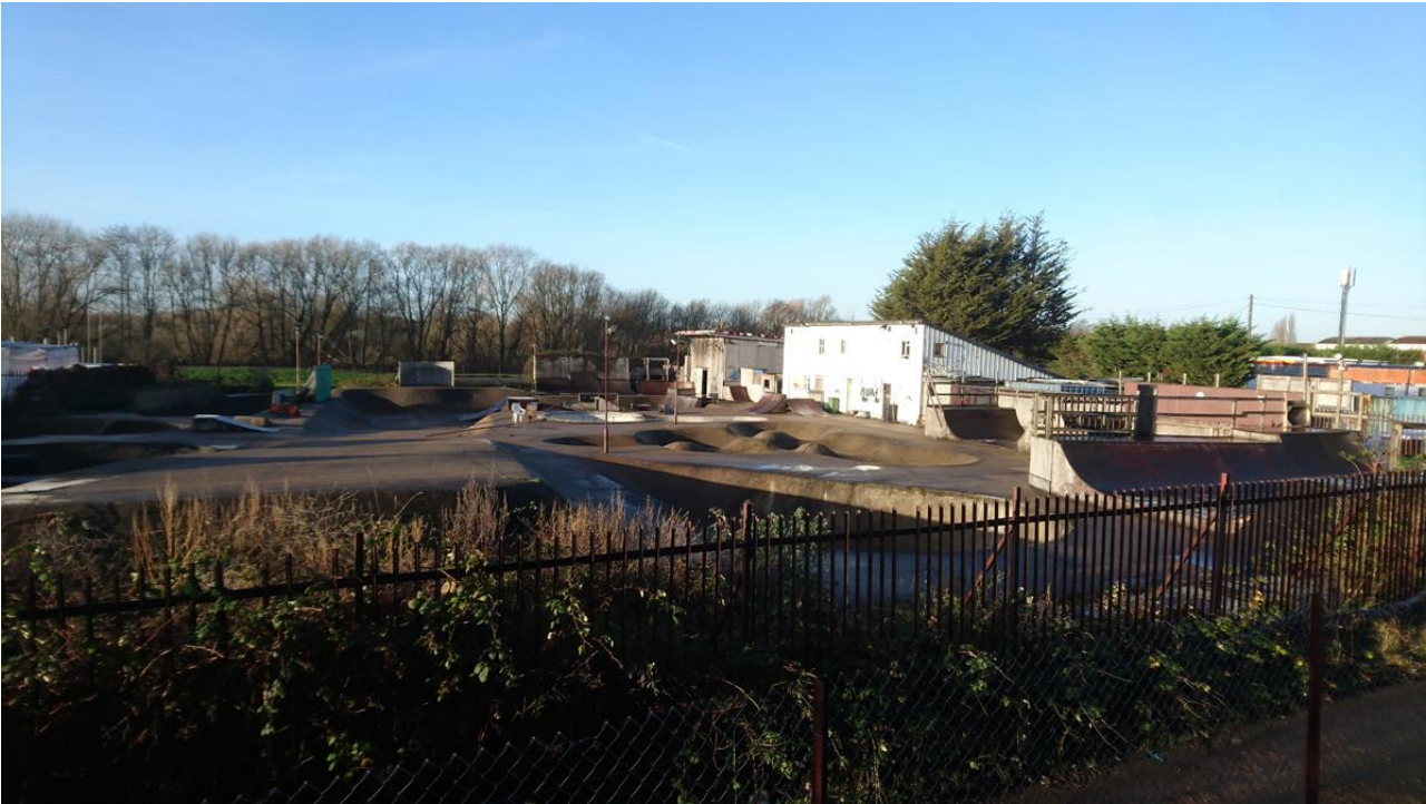
View into the south of the Site from Upper Rainham Road
