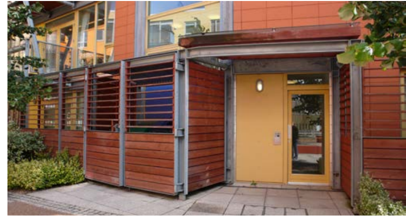
Example for well integrated communal waste and recycling storage - Greenwich Village
