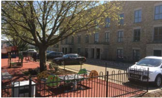
Precedent of apartment scheme - Passive House Scheme - Circle Housing on New Road
