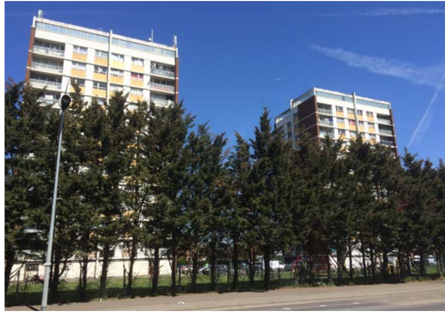
Proposals to refurbish New Plymouth and Napier House on New Road
