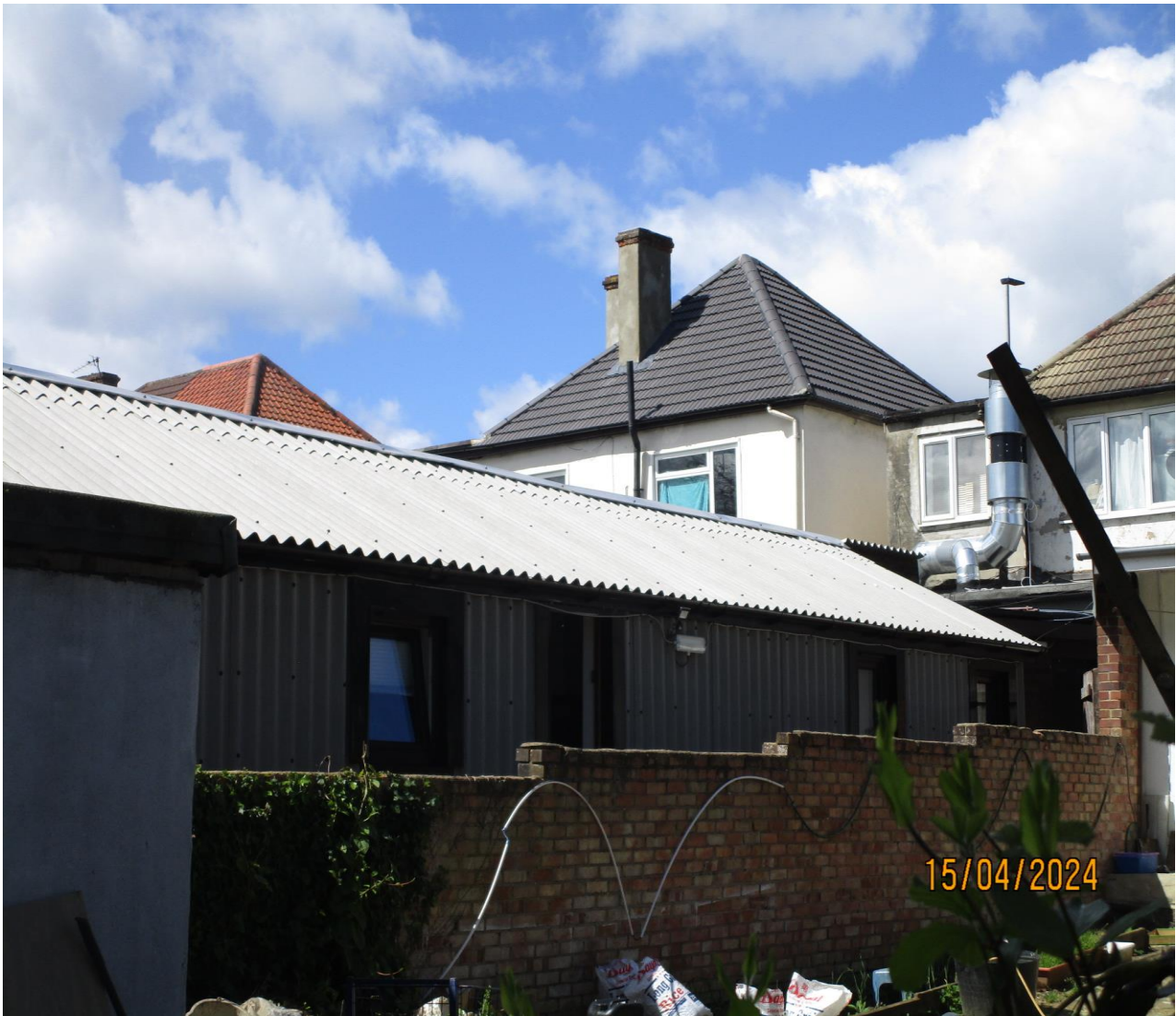
APPENDIX 1: Photo showing location of building with dwellings within rear curtilage
