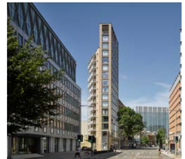
Figure 84: 67 Southwark Street, Southwark © Allies and Morrison. An example of a diminutive tower which does not dominate the skyline but makes very efficient use of a small footprint.
