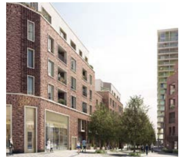
Figure 69: Agar Grove, Camden, provides a clear base, middle and crown to the building, with active frontage to the street and a stepped roofline, image © Hawkins Brown.
