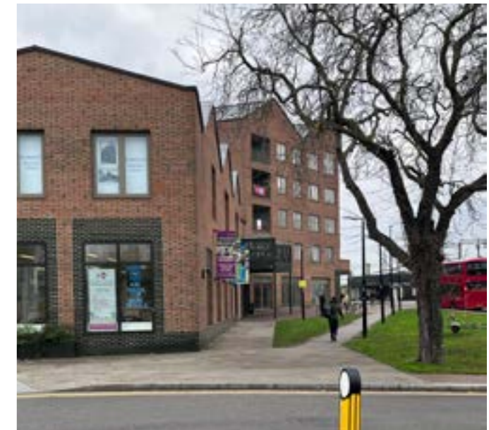
Figure 67: Development in Rainham near the station delivering a new library and homes, sensitively increases in scale from the surrounding context
