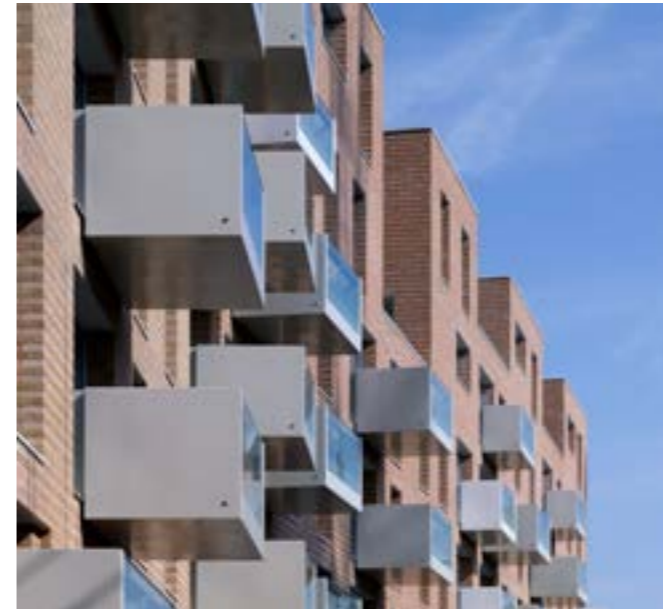
Figure 81: St Andrews, Bromley by Bow © Allies and Morrison. Mixed typology masterplan which includes courtyard blocks with taller elements as well as a standalone tower.
