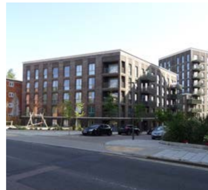
Figure 68: Lexicon in Harrow mediates between the town centre and surrounding area with a 5-11 storey scheme that has strong frontage to the main road with attractive landscaping. A good example of mid-scale high density to achieve density without towers.
