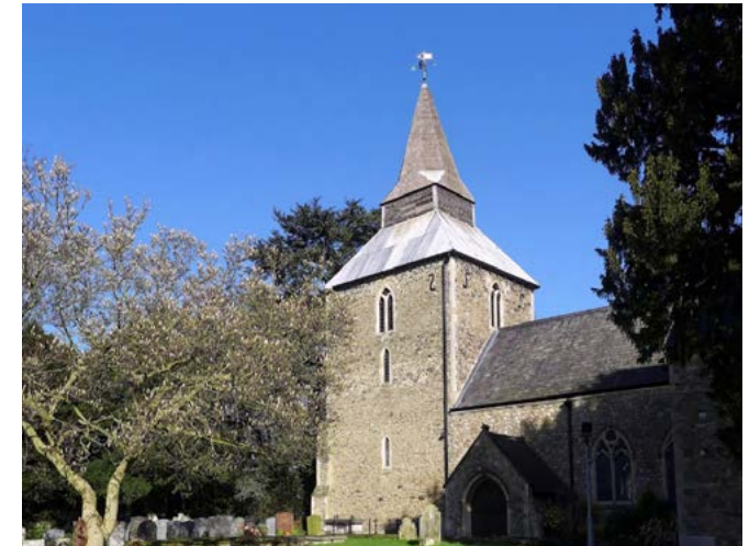
Fig 18 Source: Youtube (image to be replaced)
