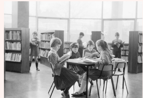
Fig 27 LB Havering Central Library, 1967 (Barking And Dagenham Archive Photos)
