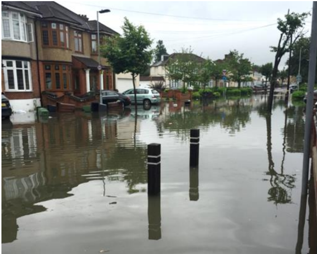
Figure 23: Photo taken by local resident taken on the morning of 23 June 16. Facing south west on Westrow Drive looking towards the junction of Manor Road and Westrow Drive showing road flooding along Westrow Drive.
