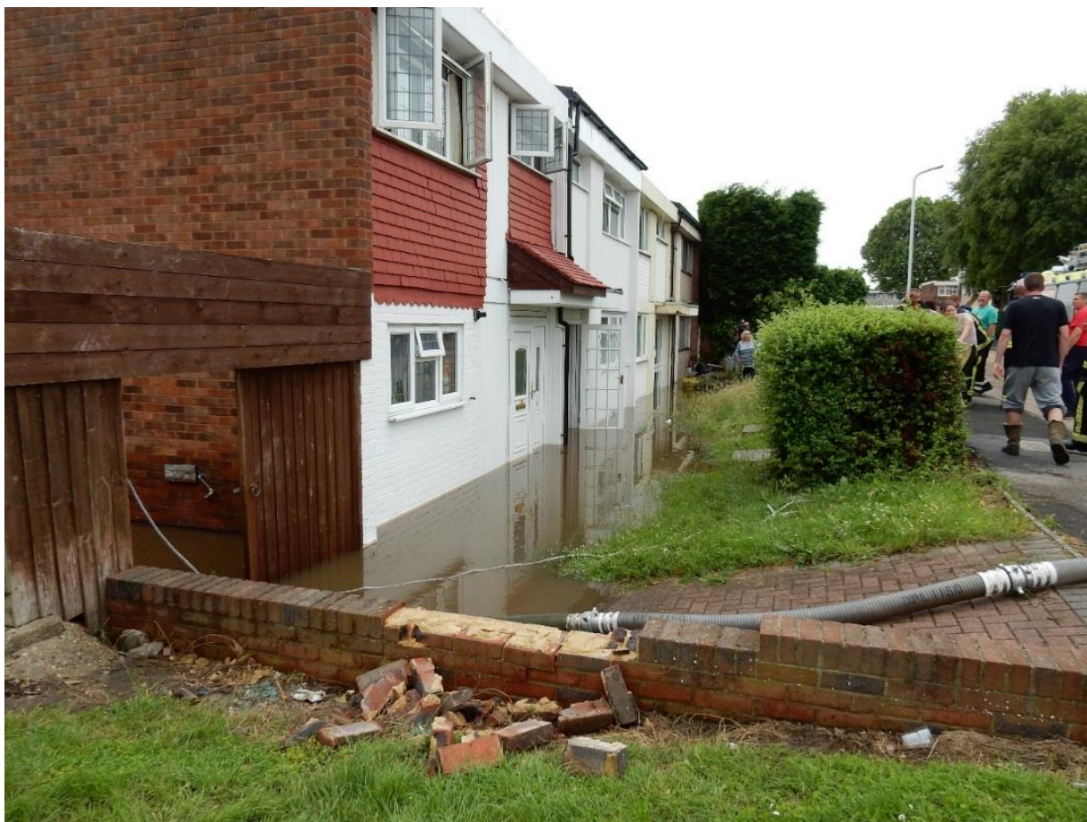
Figure 7: Photo showing properties on Penn Gardens at 12:19pm on 23 June 16. These properties had been evacuated by LFB and were being pumped out.
