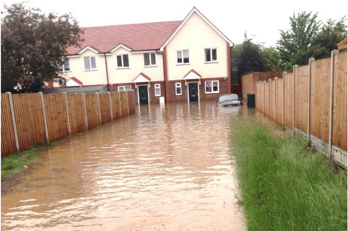
Figure 11: Photo from resident of Asten Way, showing flooded properties on Asten Way, Romford, 23 June 16
