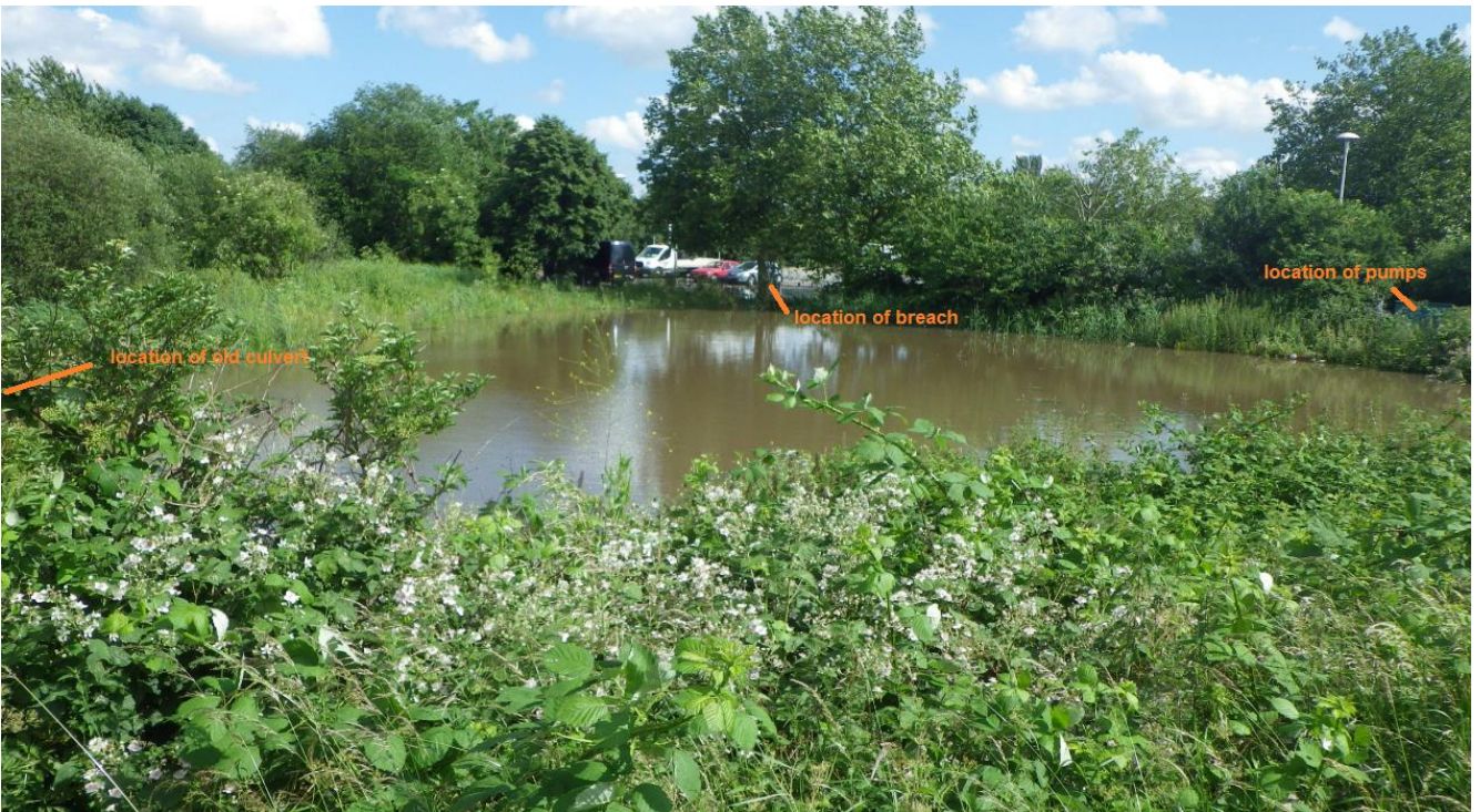
Figure 34: Photo showing Dovers Corner Flood Storage Area, 23 June 16
